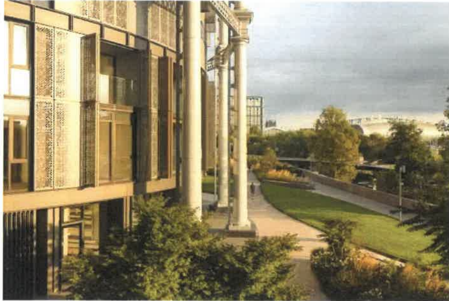
£2 million: a three-bedroom flat in Gasholders, King's Cross N1C
